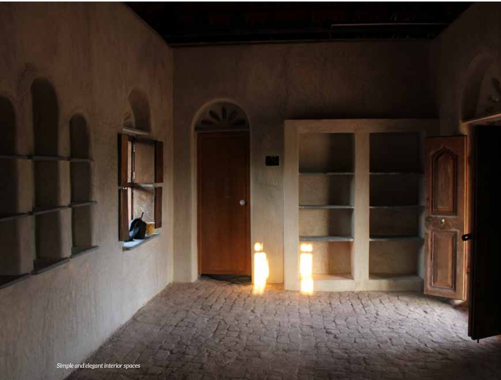
Slabs pierced into the adobe walls
